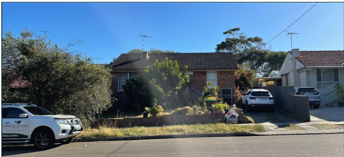
Figure 3 Development site – 48 New Orleans Crescent (Source: Site Photo, July 2023)
